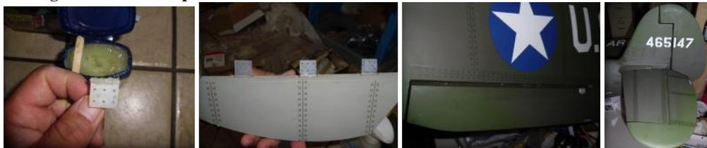
4) After the glue is completely dry on the control surface apply more Vaseline to the center of the hinge on both sides then glue the control surface with hinges into the stationary side. Press the two halves tightly together. The excess glue will come out of the center. Clean it up with Rubbing alcohol and a rag as it comes out. Work the hinge up and down a little as it's drying to help circulate the Vaseline.
